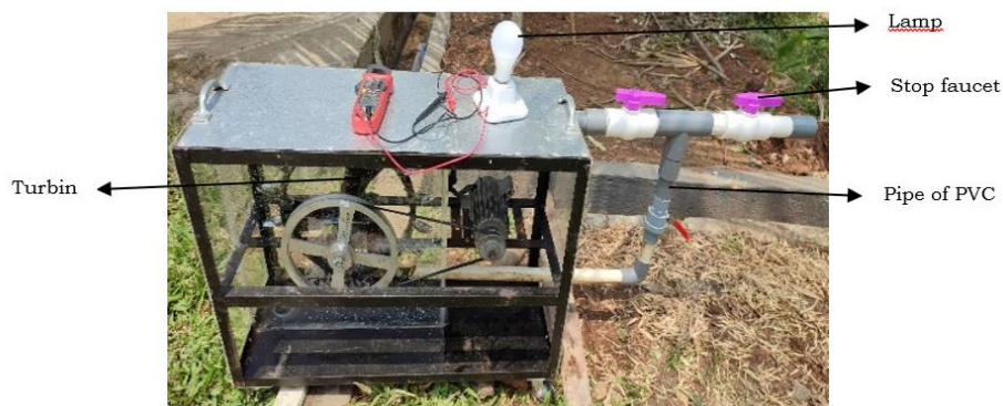
Figure 4. Suite tool installed.
